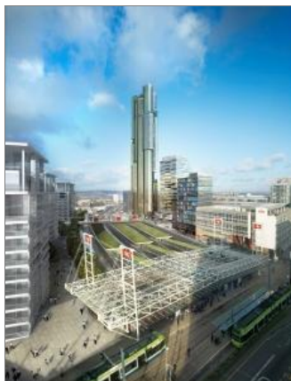
Tower with station in foreground
