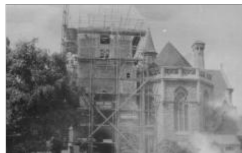
Tower under constructi on
